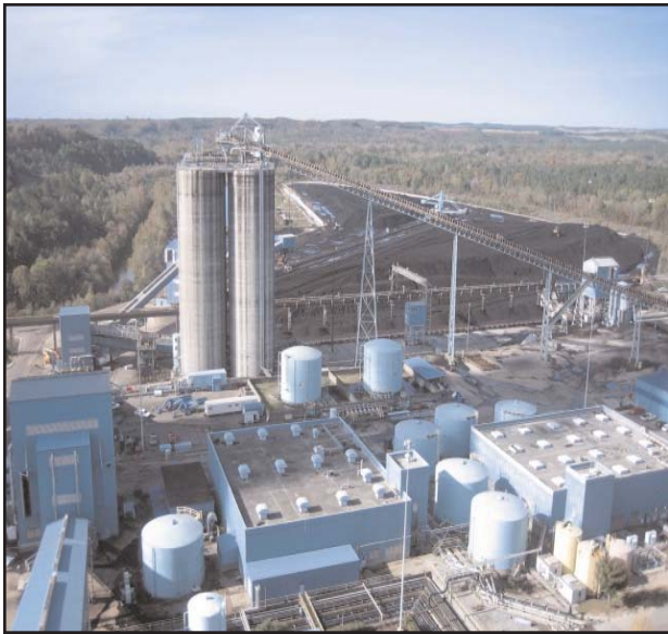
Alabama Power's James H. Miller facility
